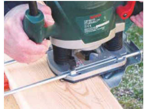
STEP 7. Rout rebates along rear edges for the matchboard. Rebates do not run full length on the side panels
